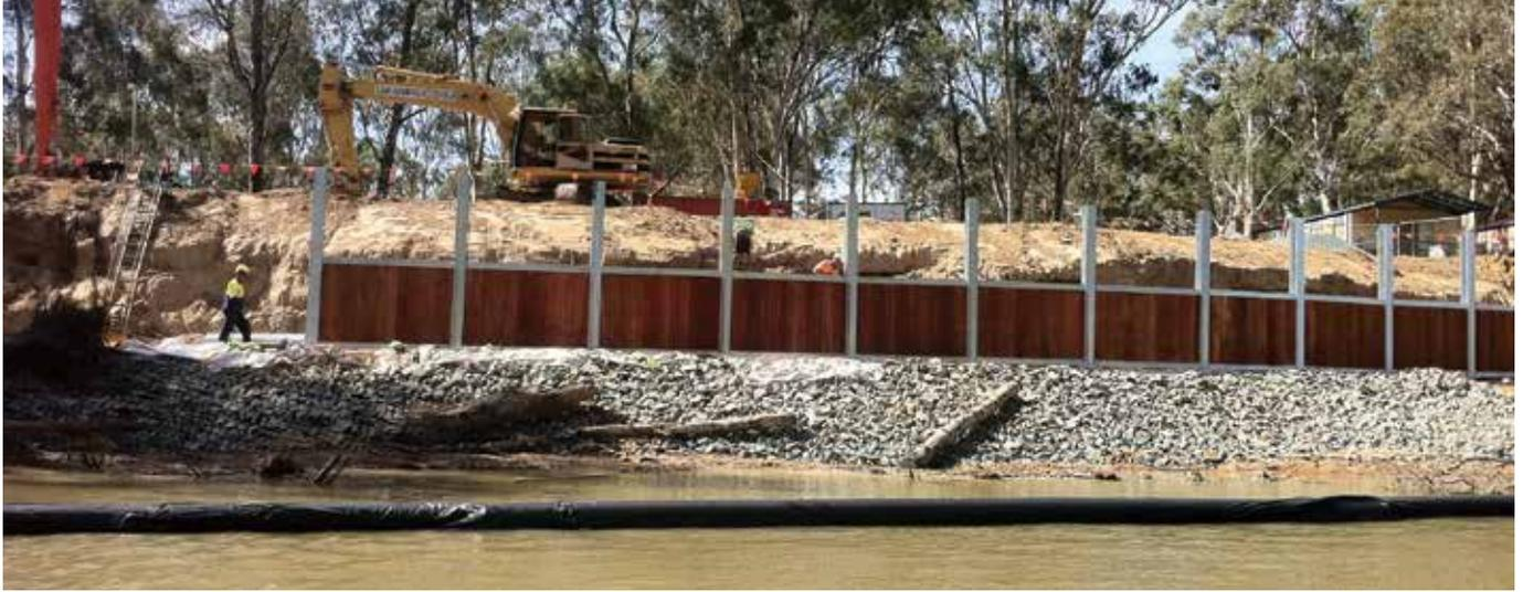
An engineered retaining wall supported by a galvanized steel frame is keeping land subsidence from encroaching on the picturesque Murray River and locals safe from floods whilst allowing red gum timber panelling to reflect the region's treasured tree life.
