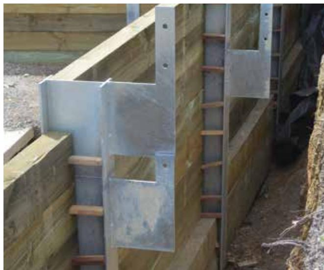
Offset fencing brackets were used to properly locate the fence on the boundary
